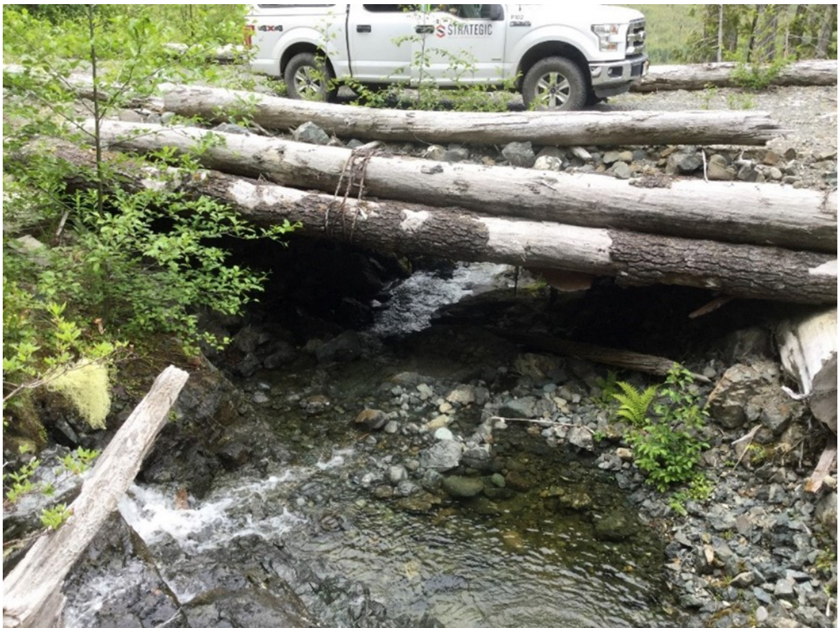
Fig 10. Today in Canada freshly felled trees are used to create a log culvert structure. Copyright CIF-IFC All Rights Reserved © 2022
