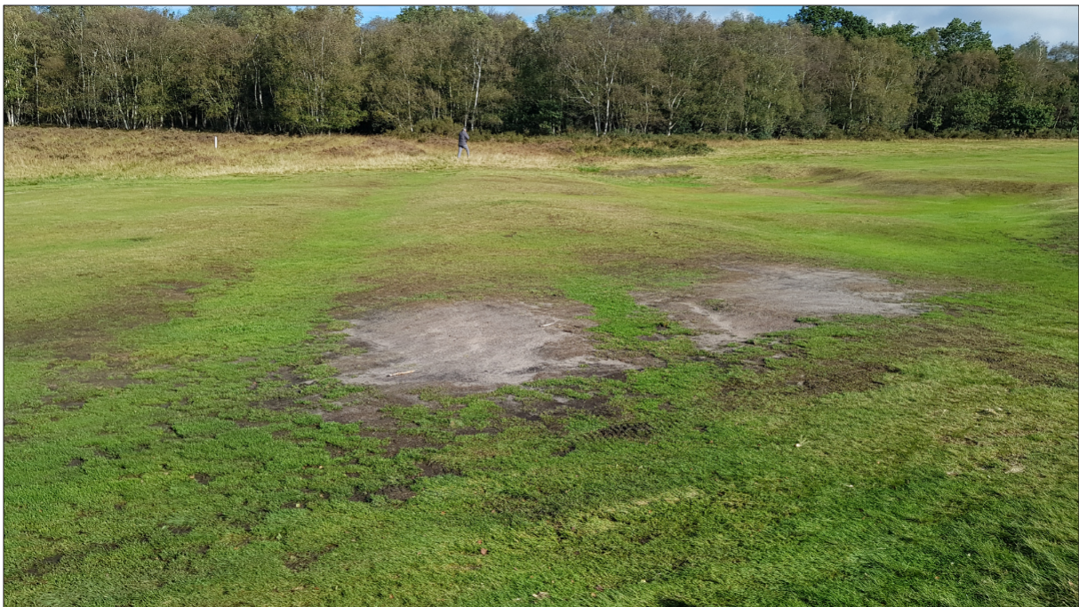
Fig. 8, Roman dual carriageway. Original agger on the left, second agger in the centre, quarry pits on the right, © K Hopkinson 2021
