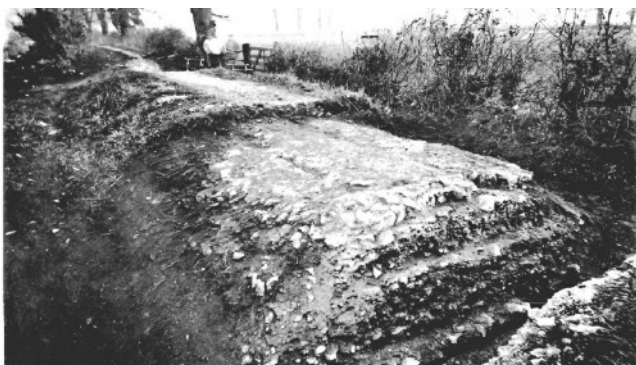
THE FOSSE AT RADSTOCK, AFTER EXCAVATION, SHOWING ITS STRUCTURAL FORMATION.
